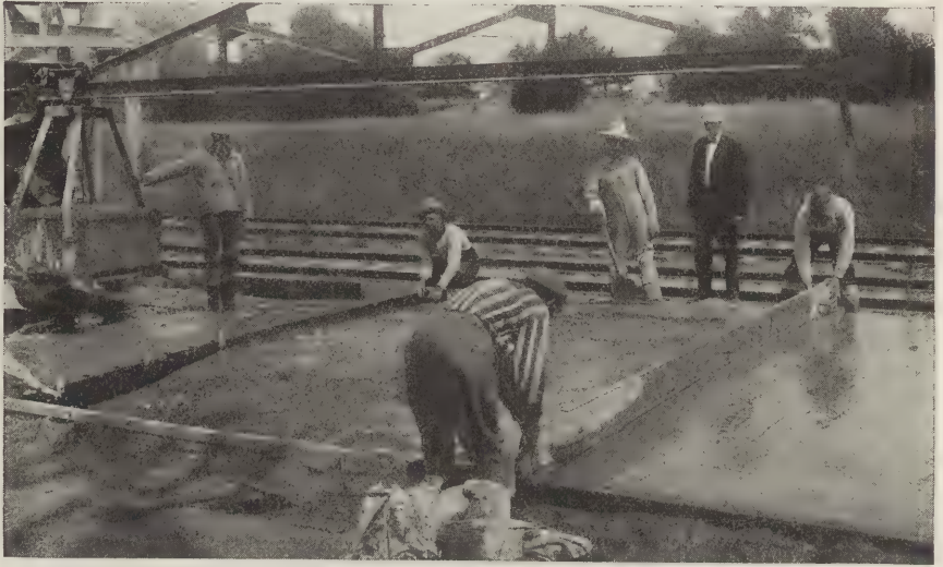
FIG. 36.—Near view of curved strike board for giving the crown to the pavement, showing also concrete bucket, mixer, boom, and steel expansion joint in place.
